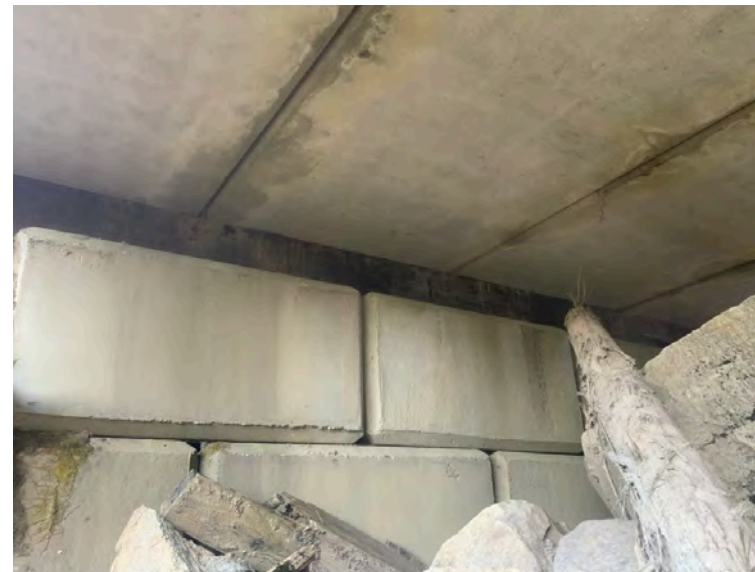
Right Bank Abutment when facing downstream
