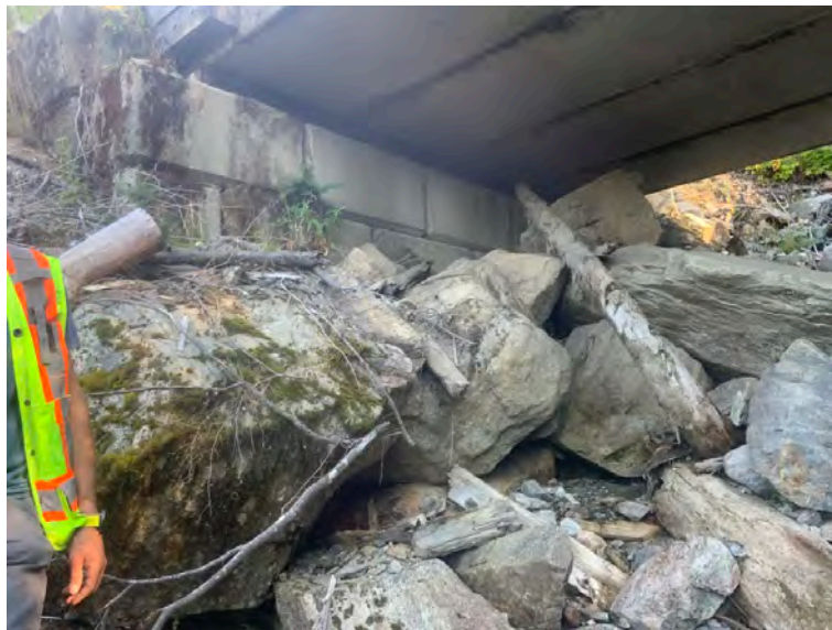
Right Bank Abutment when facing downstream
