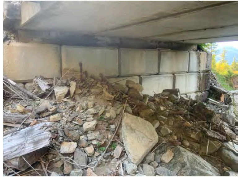
Left Bank Abutment when facing downstream
