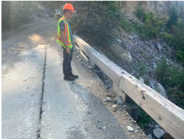
Guardrail, loose
