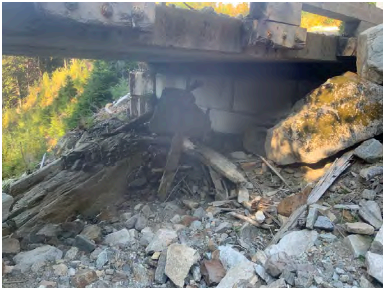
Right Bank Abutment when facing downstream
